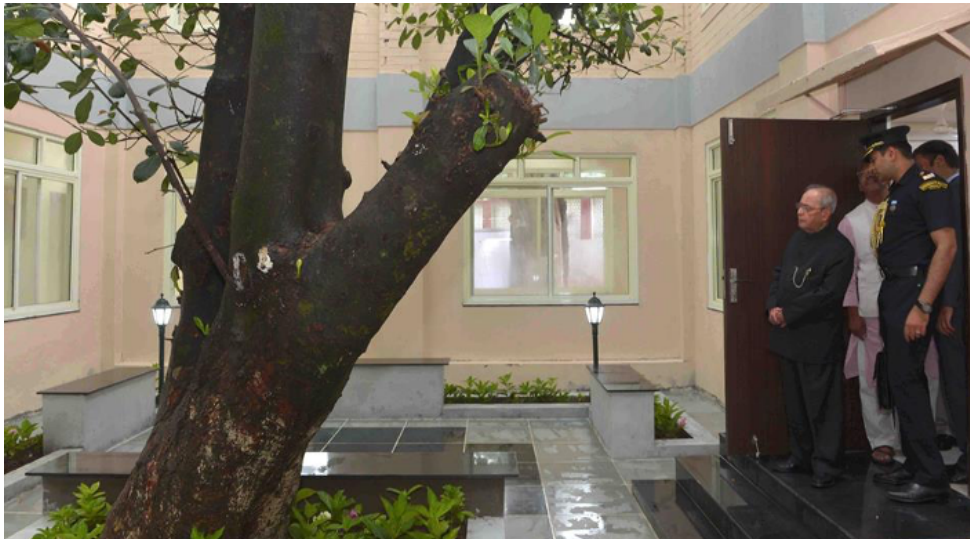
An onsite natural integrated disaster-resilient building structure deployed at the President's Estate in Dehradun, India is depicted.
